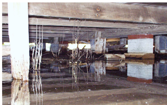
Figure 16 View to south from rear of house, showing standing water several days after rain. (NPS-SERO-CR, 2003)
