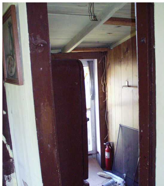
Figure 40 View to north of Room 105. (NPS-SERO-CR, 2003)
