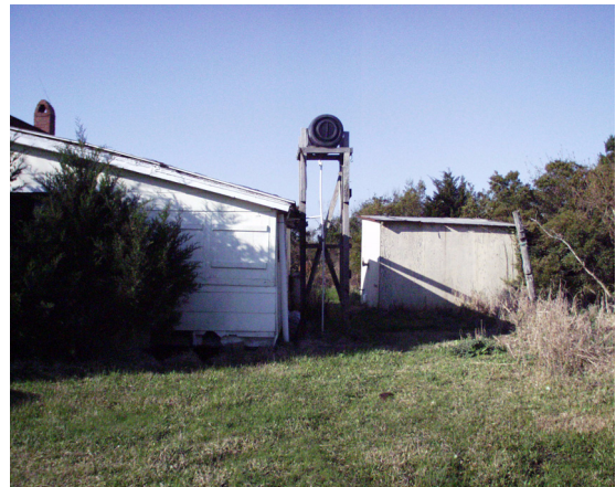
Figure 18 View southwest showing modern storage building and water tank. (NPS-SERO-CR, 2003)
