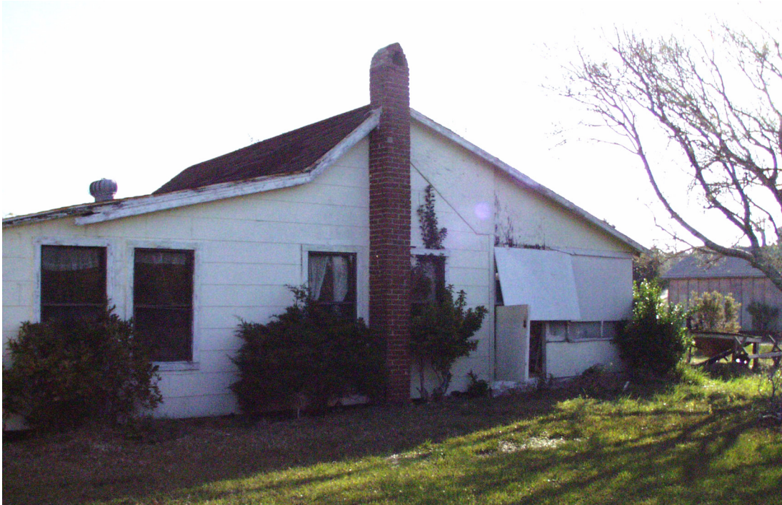
Figure 17 View east of house. (NPS-SERO-CR, 2003)
