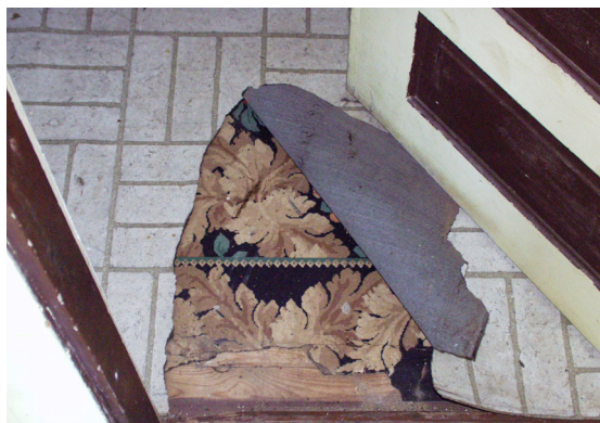
Figure 33 View of linoleum-type floor-covering underneath modern vinyl in Room 102. (NPS-SERO-CR, 2003)
